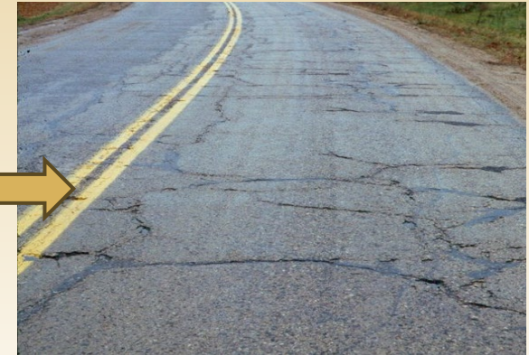
Block cracking and thermal cracking
