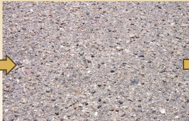
Grey and brittle material + With time – weathered surface Hot/cold temperature cycling
