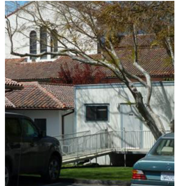
Example of a typical temporary structure
