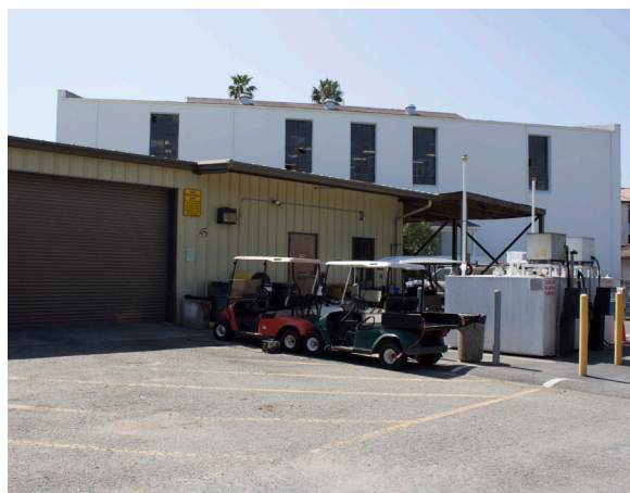
Maintenance and Vehicle Shop
