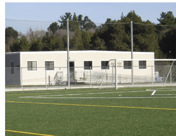
Facilities Services Building (modular)
