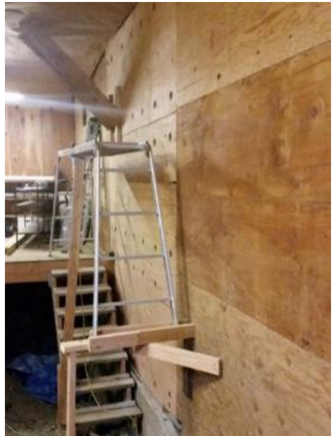
Installation of shear walls on a hillside home can help stabilize the structure during an earthquake
