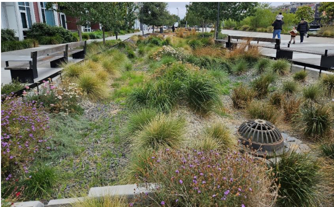
Bioswales in new development can absorb runoff and improve water quality
