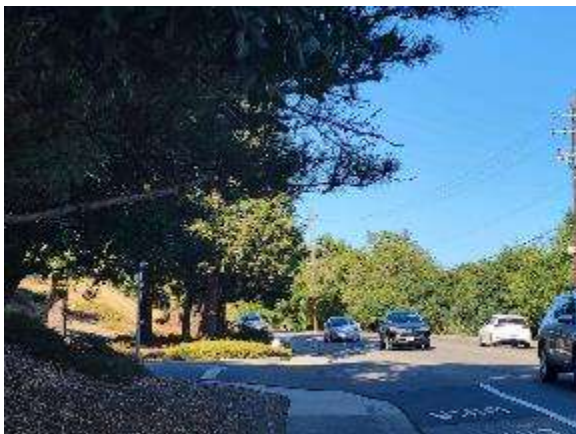
5. Moraga Road at Corte Santa Clara looking north. Impeded sightlines due to roadway alignment and trees
