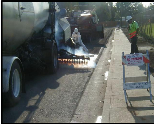
Spraying Rubber Binder Over Street
