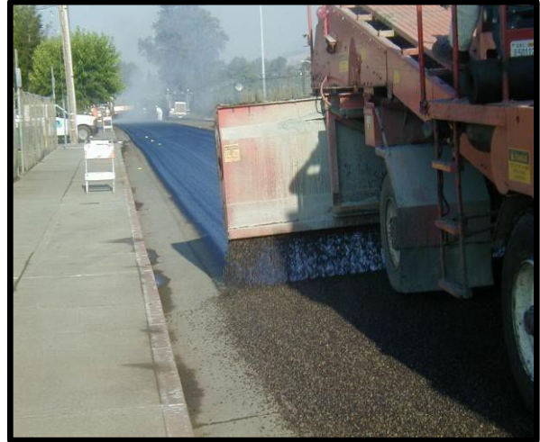
Placing Rock On Binder
