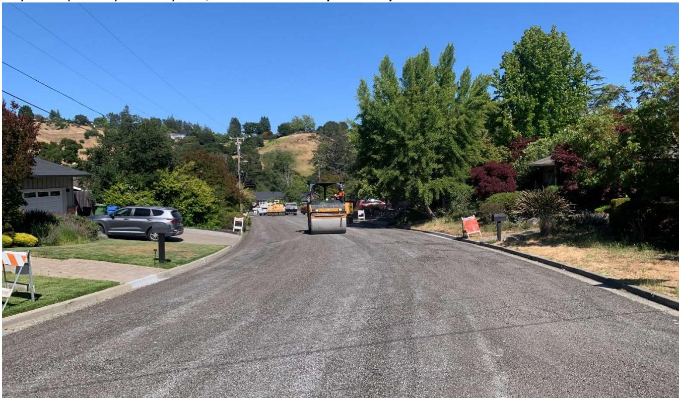
**The second component of work is applying Microsurfacing as a coating and wearing surface over the newly applied Chip Seal. When applied together, it is known as Cape Seal, and it extends pavement life substantially.**
