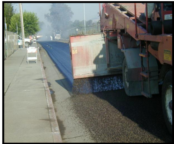
Placing Rock on Binder
