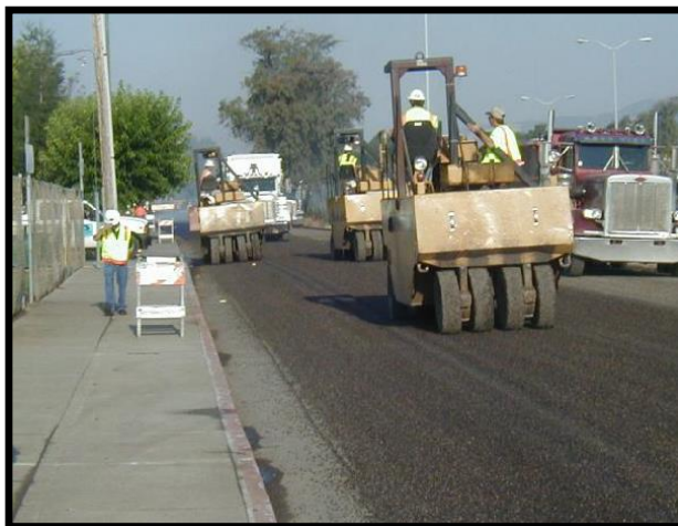
Rolling Rock into Binder
