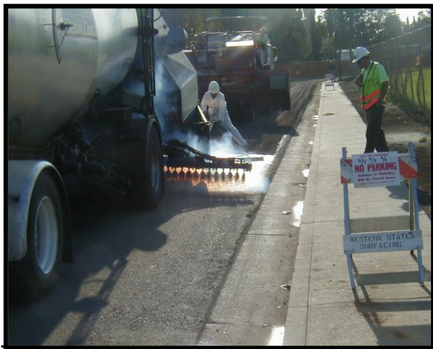
Spraying Rubber Binder Over Street
