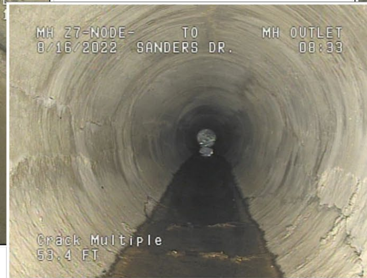
Grade 4 – Severe Cracking
