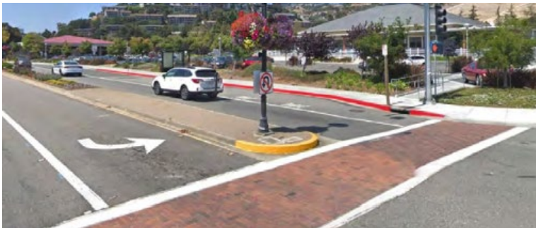
S12: Install raised median on approaches
