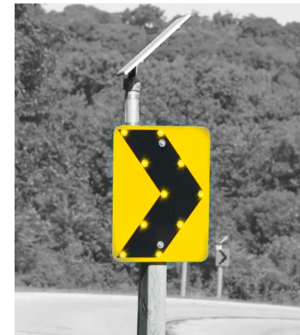
R23: Install chevron signs on horizontal curves
