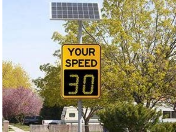
R26: Install dynamic/variable speed warning signs
