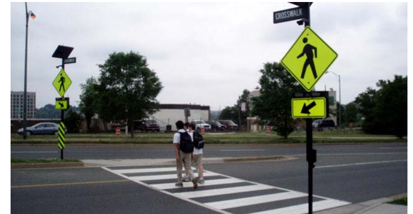
NS22PB: Install Rectangular Rapid Flashing Beacon
