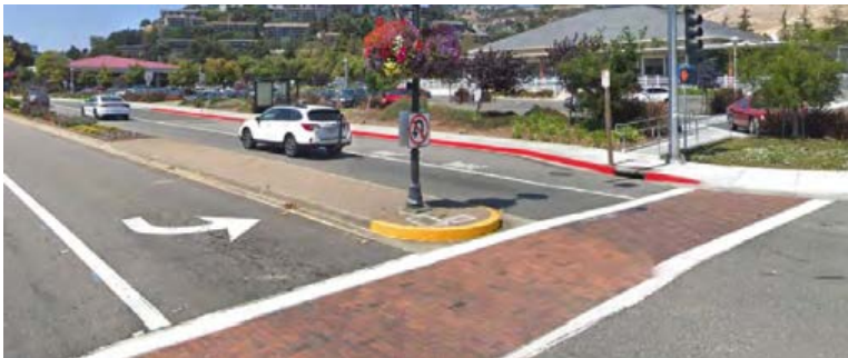
S12: Install raised median on approaches
