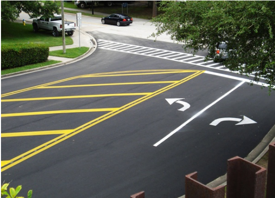
NS07: Upgrade intersection pavement markings
