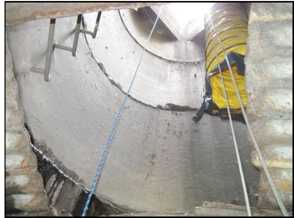
Catch Basin 14' Infiltration
