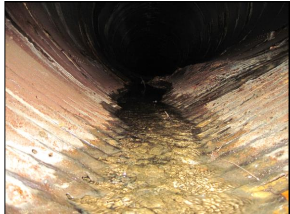
Downstream 20' Deformed (IMG_2583)
