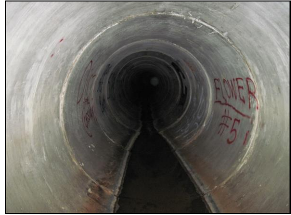
Upstream 55' Longitudinal Cracks at Joint (1)
