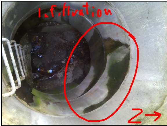
Water infiltration staining.
