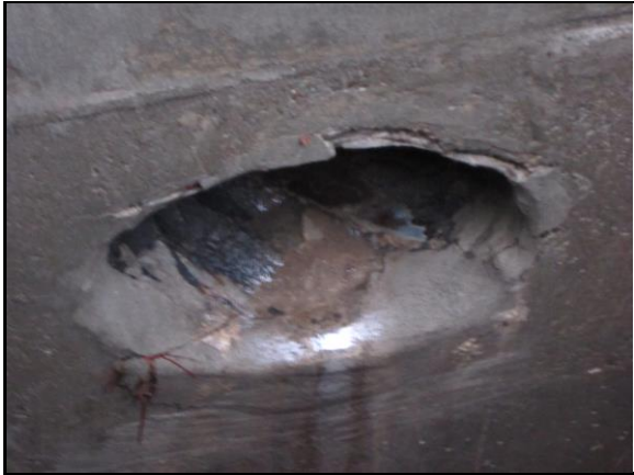
View of 16-in. CMP inlet.
