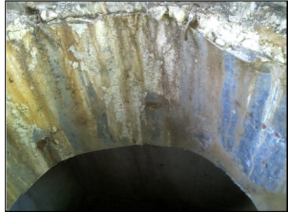
Delaminating metal lining on manhole chimney.
