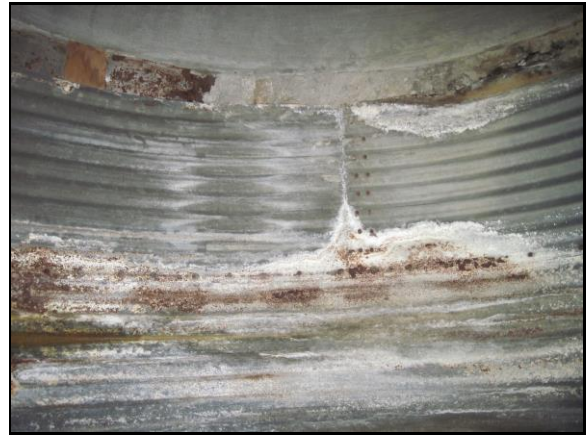
Upstream 46' Defective Pipe Material Change (1)
