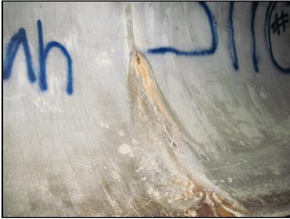
Upstream 73' Longitudinal Cracks, Staining (1)
