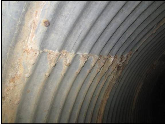
View of encrustation on pipe wall.
