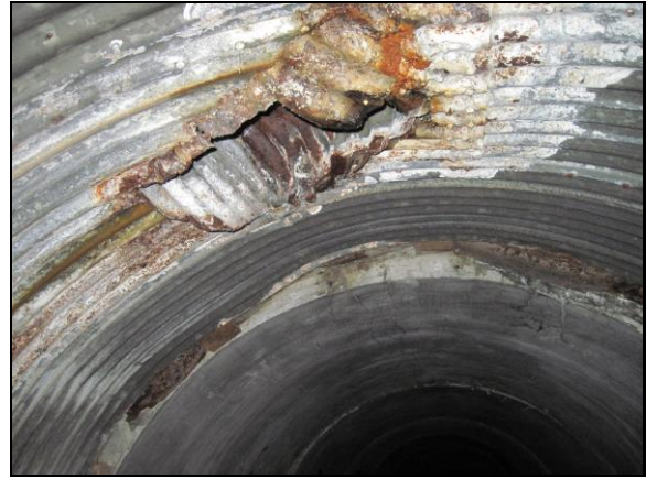
Upstream 45.5' Defective Tap Connection (1)
