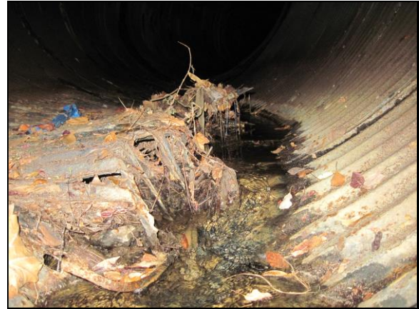
Upstream 8' Broken Pipe (1)
