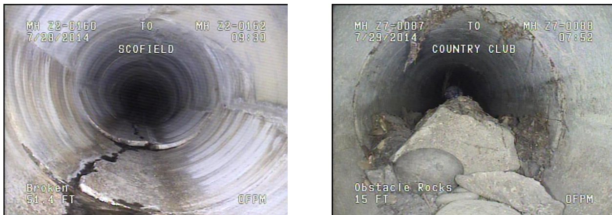
Figure 2: Pipe Impairment Examples: Broken Pipe (left) Pipe Debris (right)
