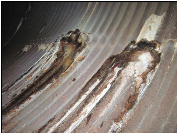
Downstream 3' Infiltration (1)
