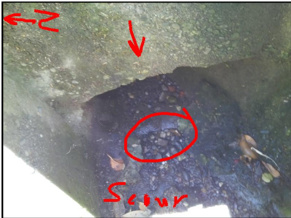
View of inlet. Scouring on structure floor.
