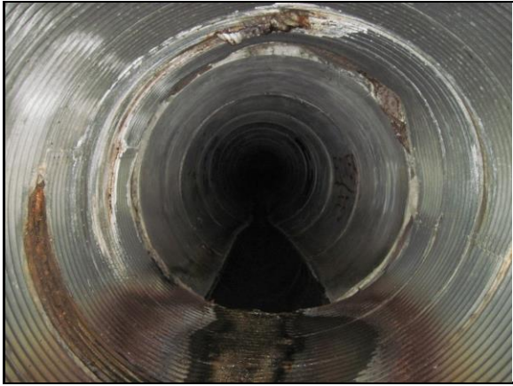
Upstream 46' Defective Pipe Material Change (4)
