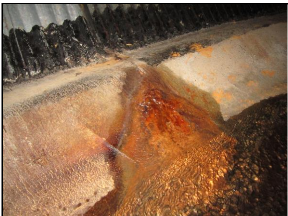
Infiltration staining.
