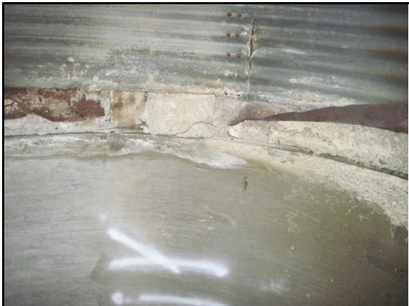
Upstream 46' Defective Pipe Material Change (2)
