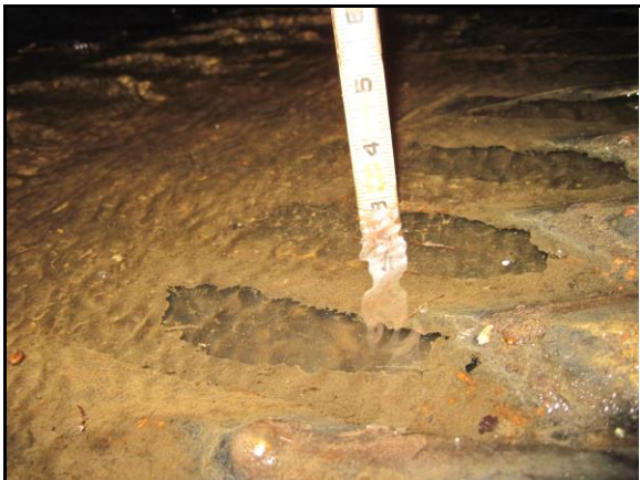
Downstream 411' Hole Void Visible (IMG_2654)
