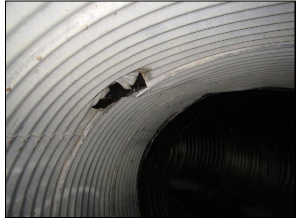
Hole in pipe wall.
