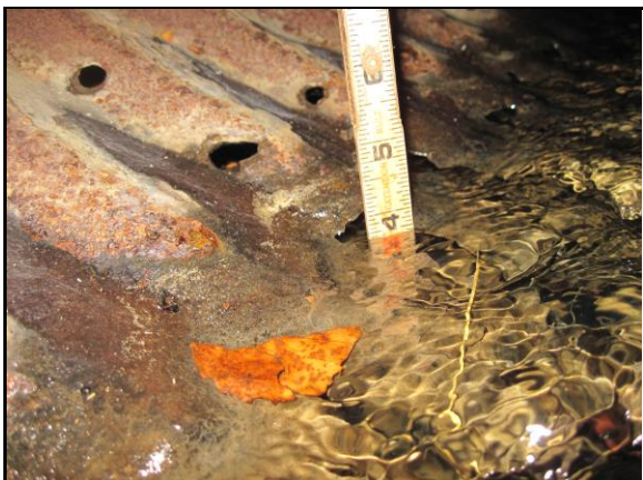
Downstream 20' Holes Void Visible
