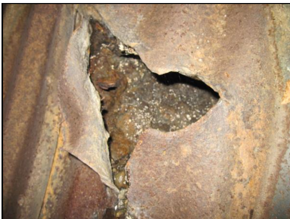
Upstream 8' Hole Void Visible (1)
