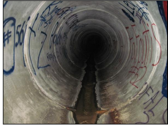
Upstream 81' Longitudinal Cracks, Staining (3)
