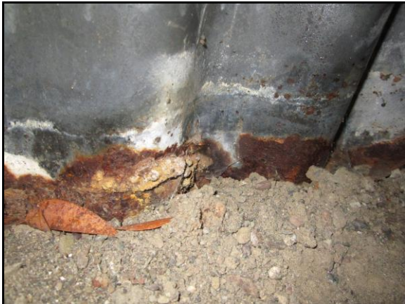
Corrosion on pipe wall.
