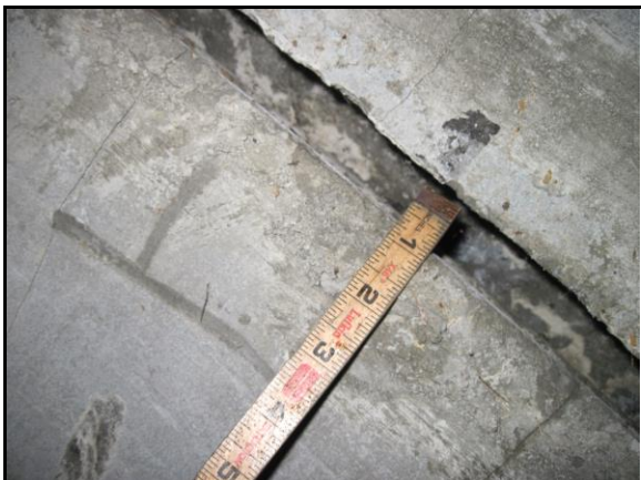
Upstream 65' Missing Mortar (2)
