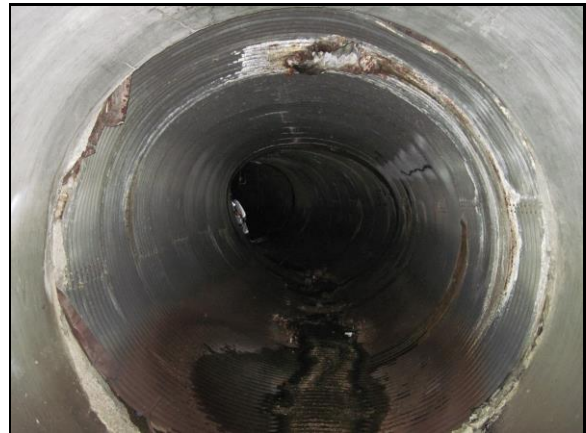
Upstream 46' Defective Pipe Material Change (3)
