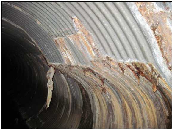
Downstream 207' Deformed (1)
