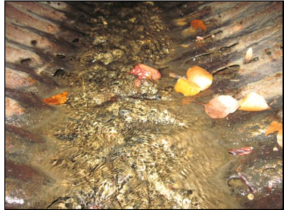
Downstream 13' Holes Void Visible
