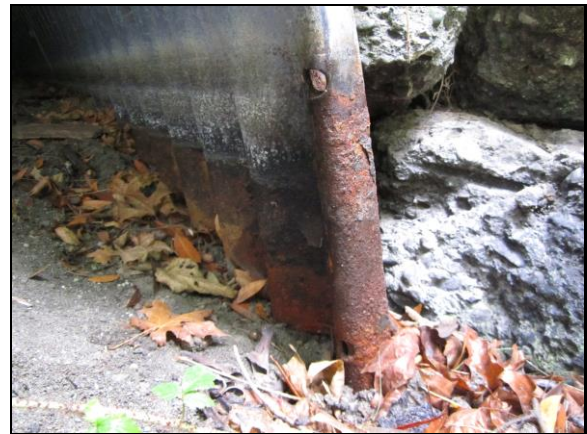
Corrosion on pipe wall.
