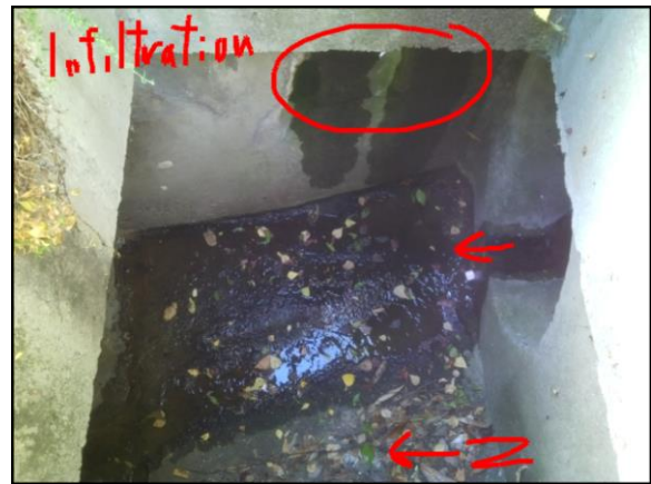
Down view of structure. Water infiltration staining.
