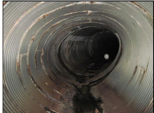
Upstream 18' Deformation
