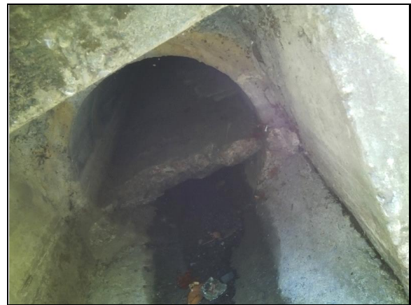
View of outlet. Concrete slab obstructing pipe.
