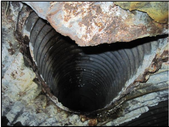
Upstream 45.5' Defective Tap Connection (4)
