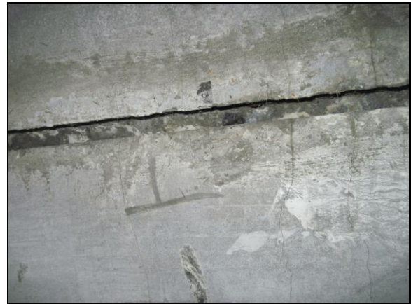
Upstream 65' Missing Mortar (1)
