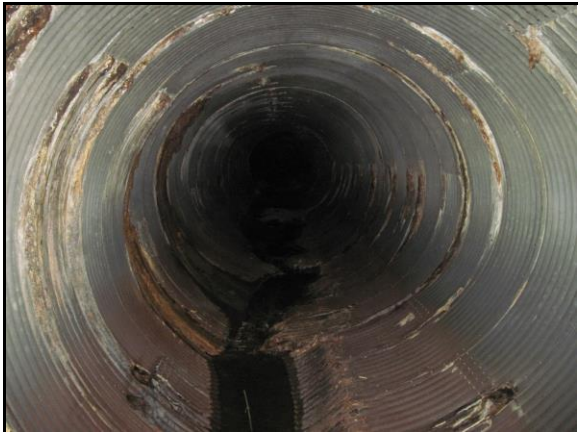
Downstream 20' Deformed (IMG_2580)
