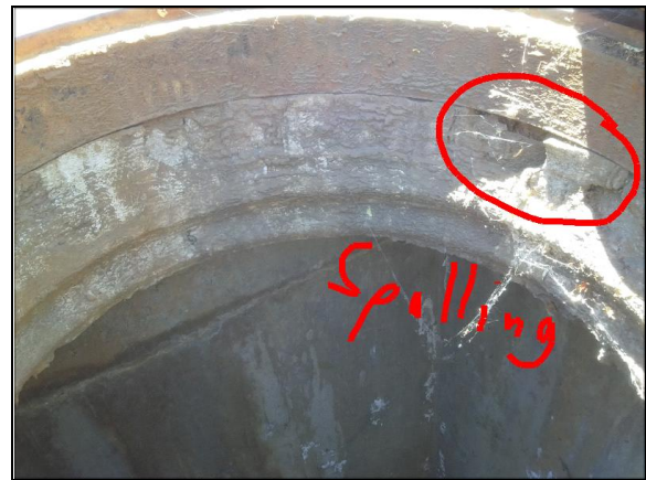
View inside manhole. Spalled concrete on manhole chimney.
