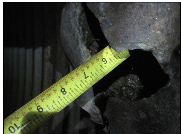
Upstream 8' Hole Void Visible (2)
