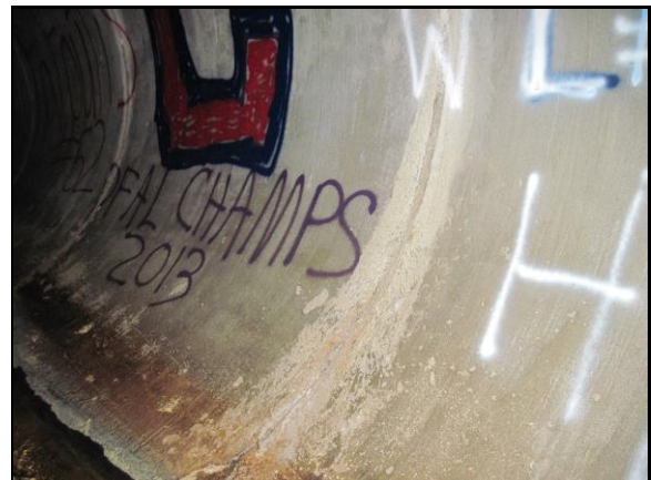
Upstream 73' Infiltration Stains
