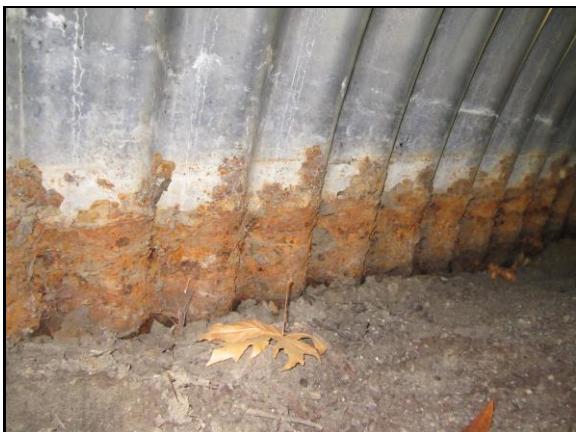
Corrosion on pipe wall
