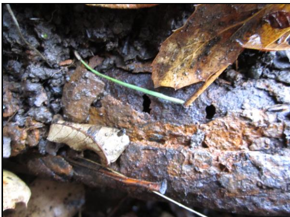
Minor perforations in pipe crown at inlet.
