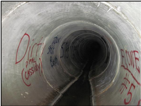
Upstream 55' Longitudinal Cracks at Joint (2)
