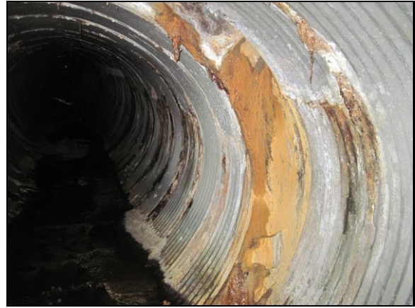
Downstream 77' Defective Pipe Size Change (2)
