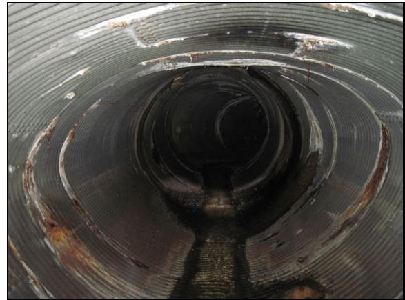
Downstream 337' Deformed
