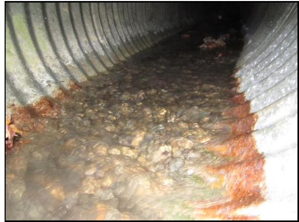
View of invert of nearby 30-in. CMP outlet.
