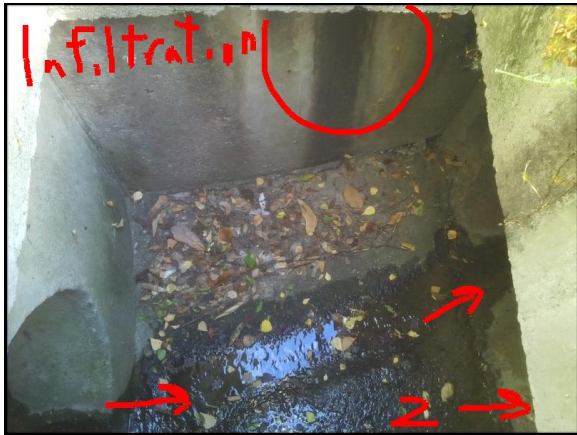
Down view of structure. Water infiltration staining.
