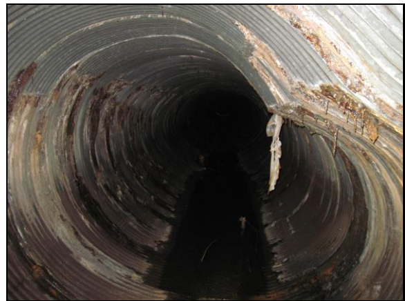
Downstream 207' Deformed (2)
