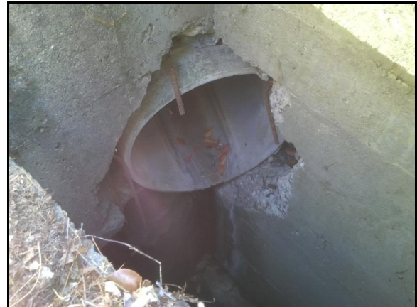
Projecting reinforcing steel and exposed aggregate.
