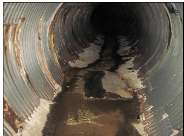
Downstream 40' Patch Repair
