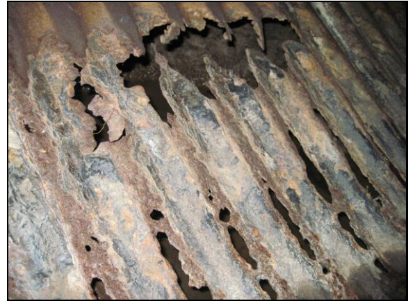
Upstream 15' Hole Void Visible
