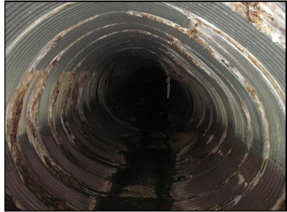
Downstream 186' Deformed (IMG_2636)
