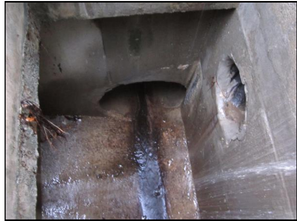
View of 36-in. RCP outlet and 16-in. CMP inlet.
