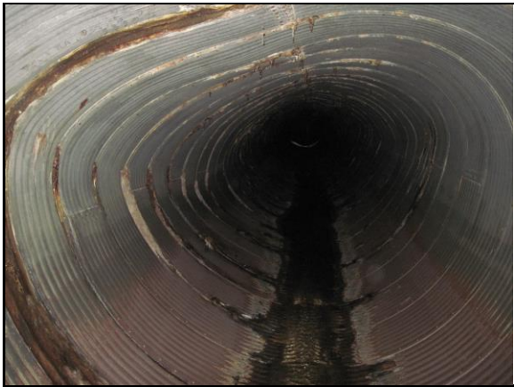
Downstream 270' Deformed (IMG_2644)
