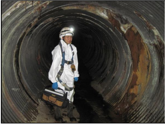
Downstream 77' Defective Pipe Size Change (1)
