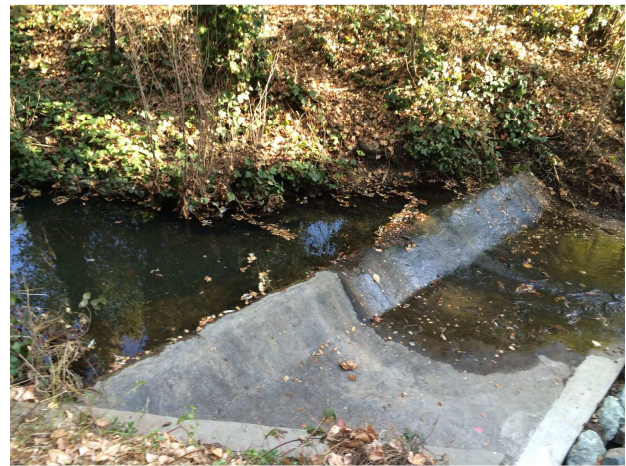
Photo 2. Concrete Spillway Apron
