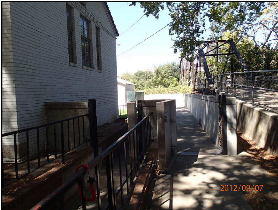
Photo 16. Floodwall Gate at the Roseville Veterans Memorial Hall
