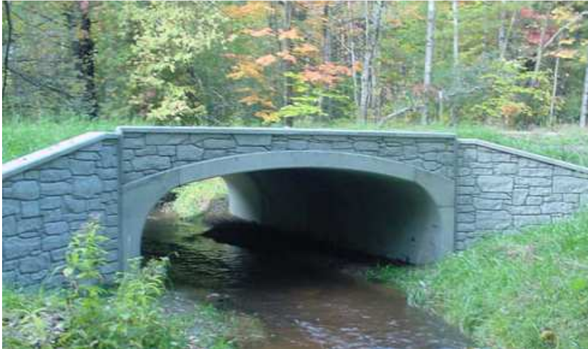
Photo 20. (Left) Sickie Creek Precast Concrete Arch with Wingwalls
