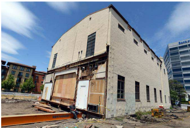
Photo 9. Inserting I-Beam below Masonic Temple
