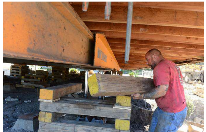
Photo 10. Hydraulic Jack used to Lift the Masonic Temple
