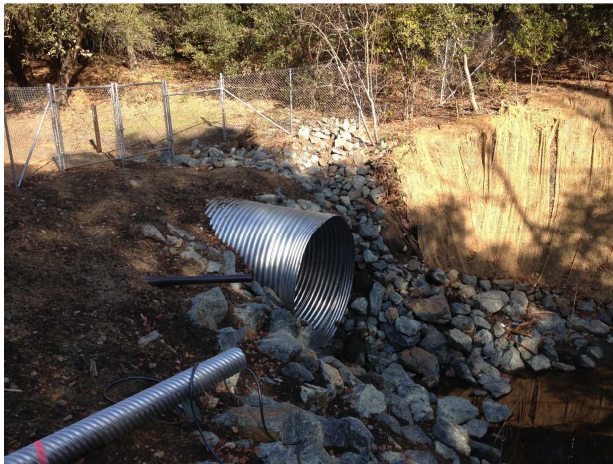
Photo 4. Downstream Face of the Existing 8-ft CMP Culvert
