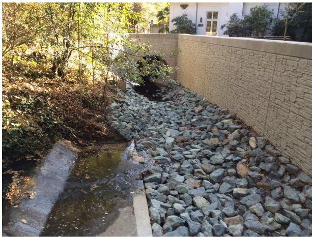
Photo 1. Upstream of Existing 8-ft CMP Culvert
