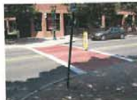
Transverse Crosswalk with Colored Pavement
