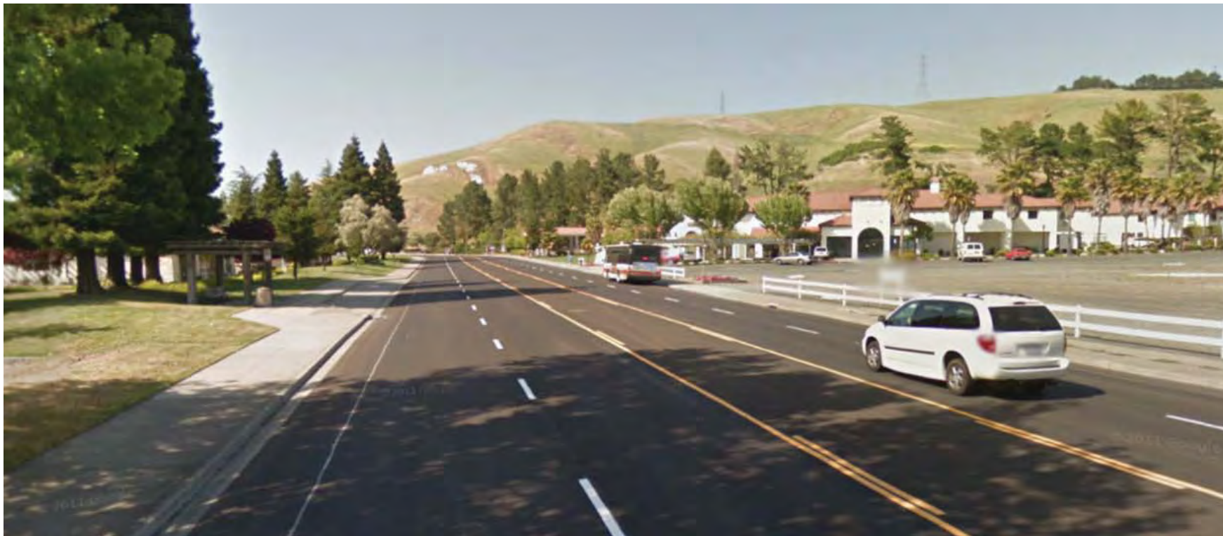
Looking north, approaching Rheem Boulevard.
