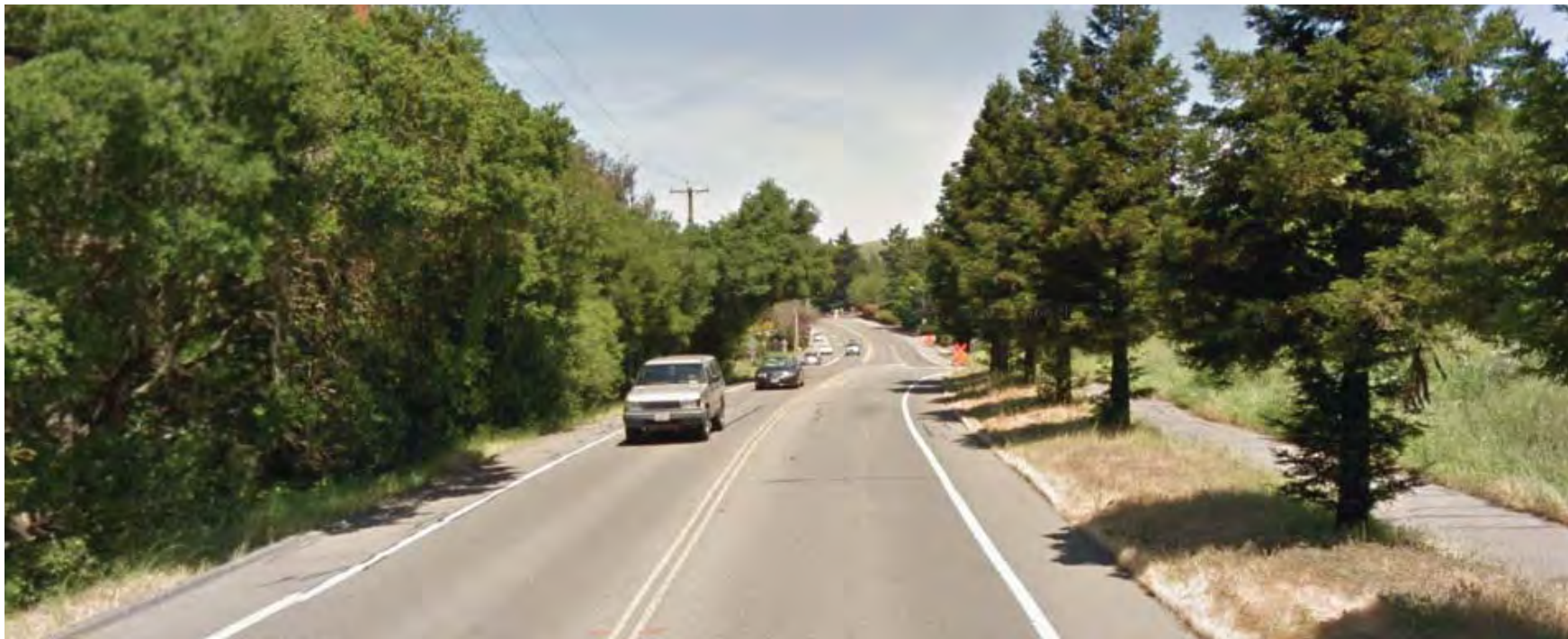
Looking North on Moraga Road, approaching Corliss Drive.
