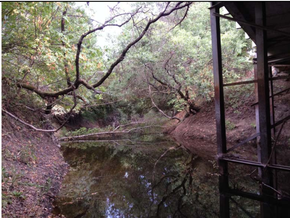
Moraga Creek (PD 1) at Canyon Road crossing facing southwest. Photograph date: July 15, 2014.
