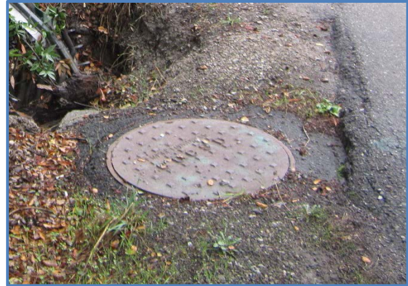
Figure 2-4. Storm Drain Inlet (left) Storm Drain Manhole (right)
