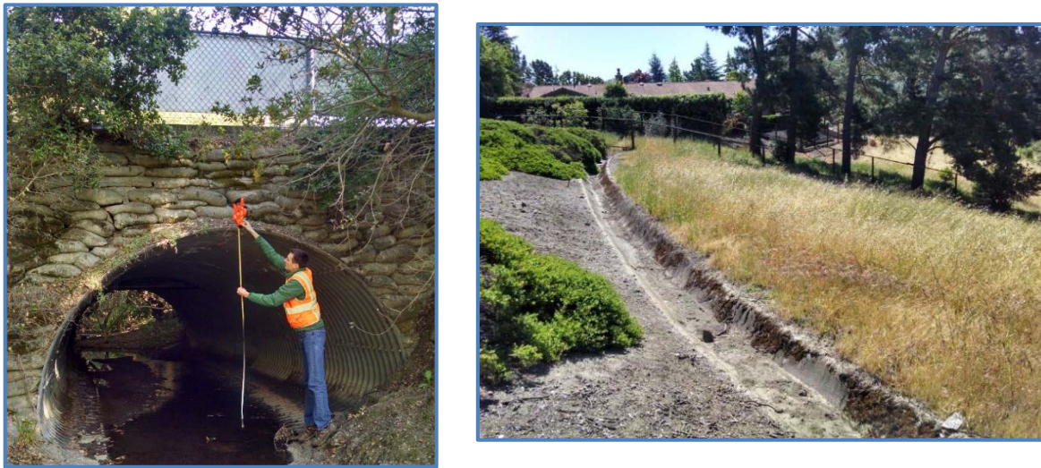
Figure 2-3. Creek Culvert (left) and Concrete Lined Ditch (right)
