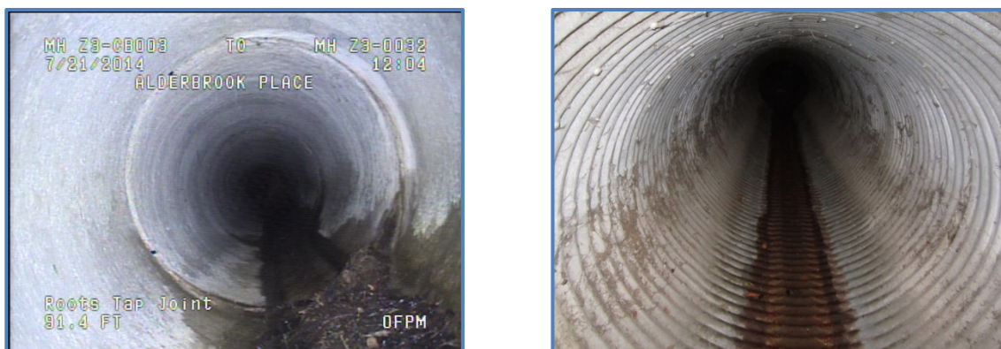
Figure 2-1. Typical Public Storm Drain Pipes – RCP (left) and CMP (right)
