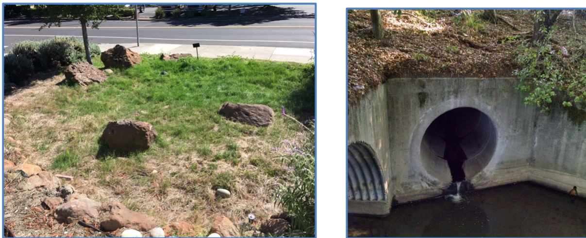
Figure 2-5. Bioretention Basin (left) Storm Drain Outfall (right)
