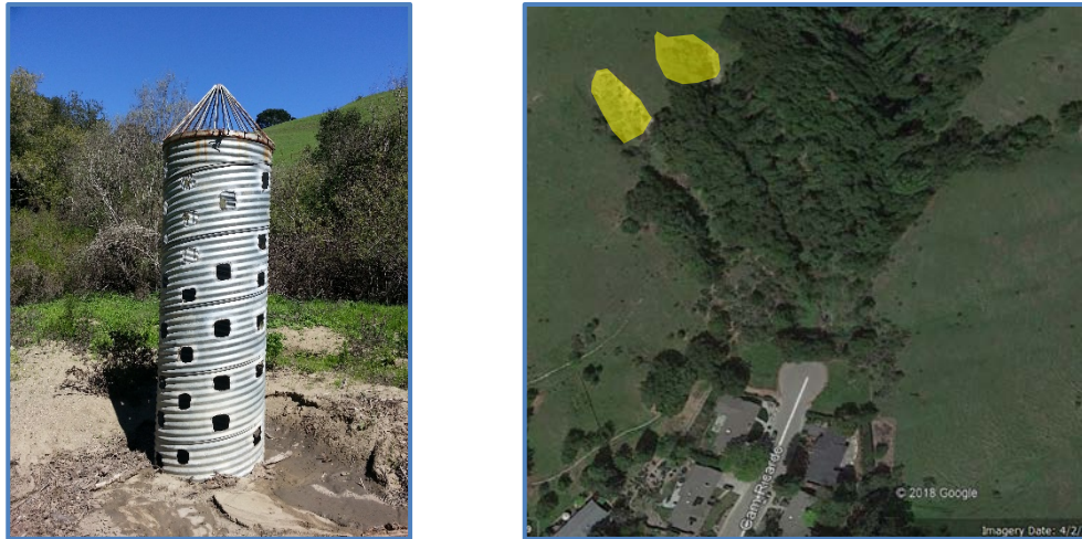
Figure 3-1. Missouri Riser Structure (left) Active Landslide Areas in Yellow (right)
