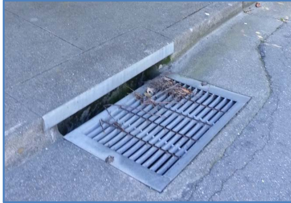
Figure 2-4. Storm Drain Inlet (left) Storm Drain Manhole (right)
