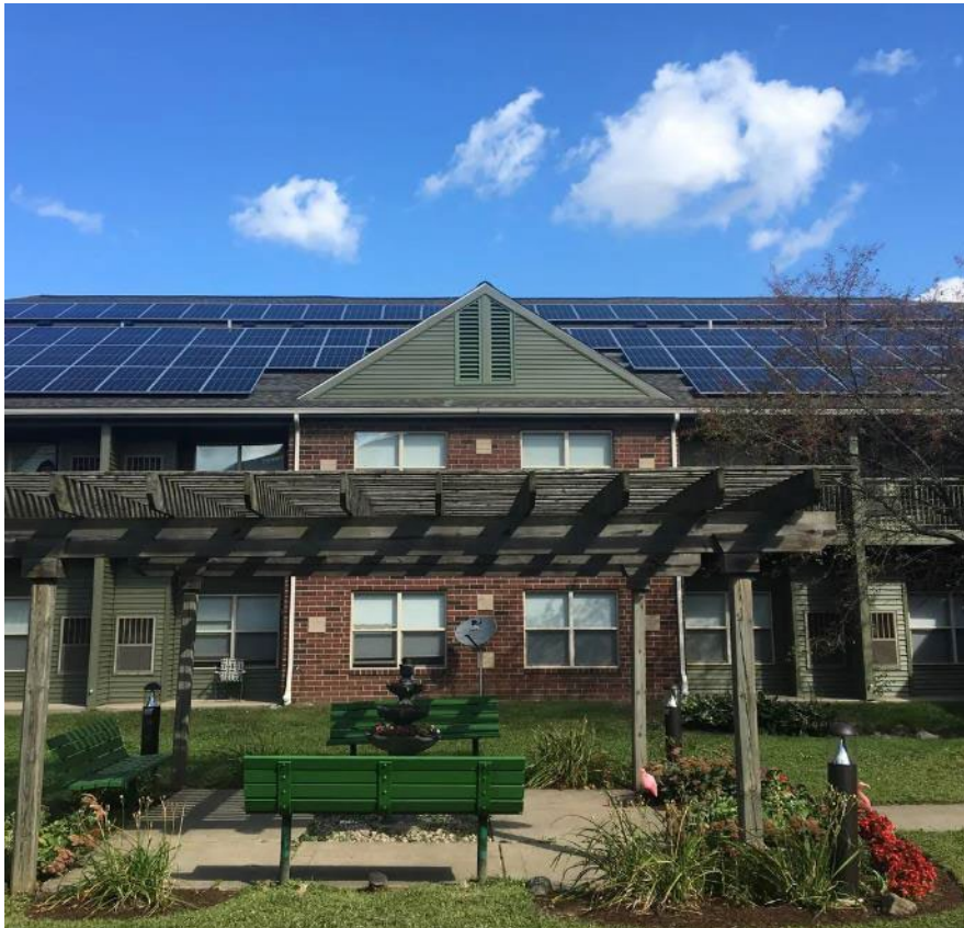
Roof mount solar on angled roof
