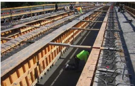
The Canyon Road Bridge Replacement Project is in its twelfth week of construction. The July 3 early morning mass concrete pour of the stem, soffit, and abutments was a success. In the next two weeks, the contractor will form and pour the bridge deck. We appreciate everyone's patience and cooperation. For more information, please visit the [Project website](#) page. To sign up for project updates, please register at [Notify Me](#)
